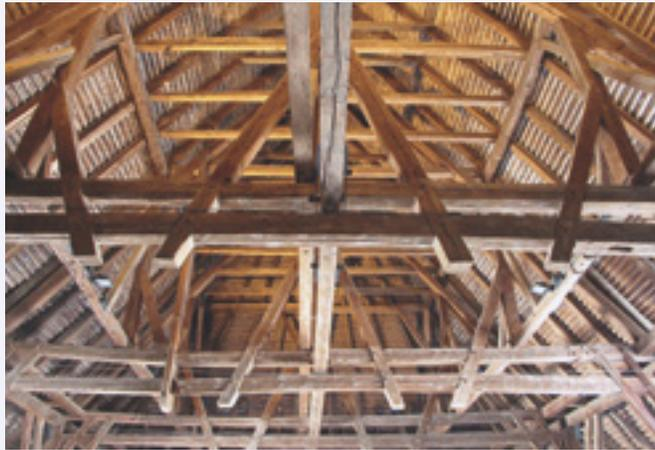
The Old Builders Yard in the Franconian Open Air Museum was built in 1443. The roof timbers span 350 m<sup>2</sup> without the use of a single support – a superb technical achievement.
