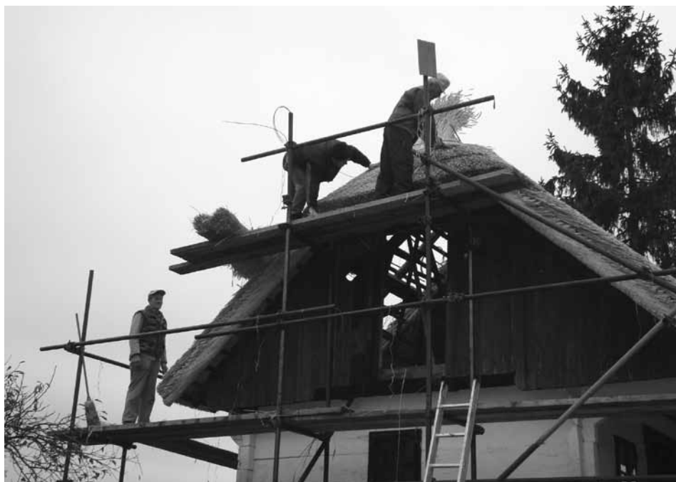
Prekrivanje krovova slamom Covering of the roofs by straw
