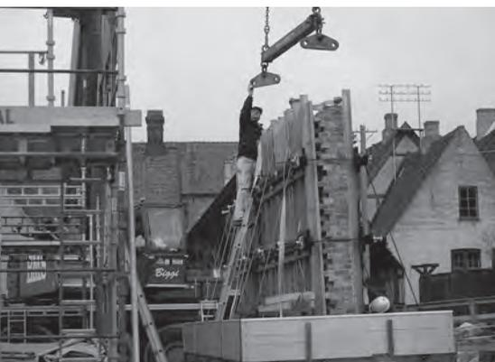
January 2011. The first brick-section of the Hjørring-house is craned to its permanent position.
